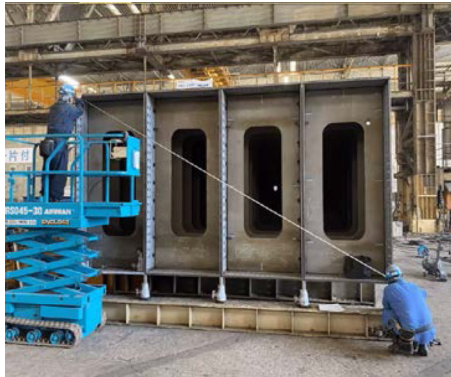
(a) Fabrication of reaction beam
